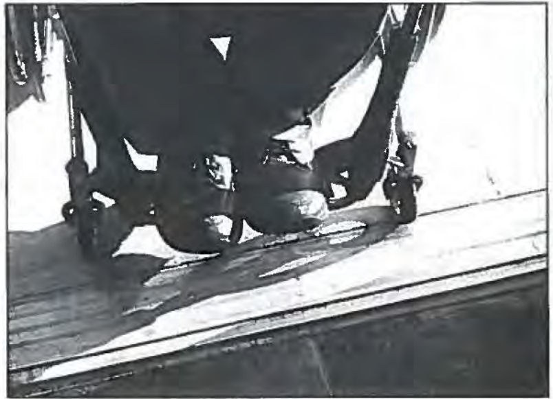
Figure 9: Low profile door threshold Photo by Ron Wickman
