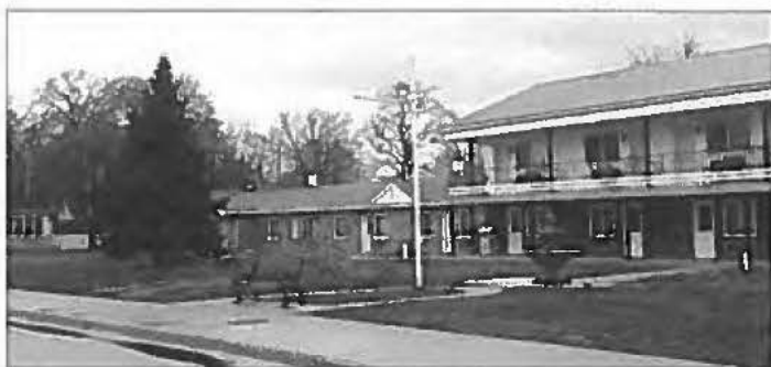
Figure 1 Blue Haven Apartments in Amherstburg, Ontario
