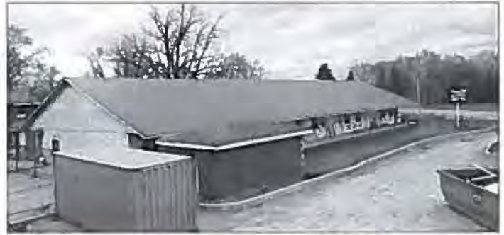
Figure 2 Blue Haven Motel under renovation to affordable housing
